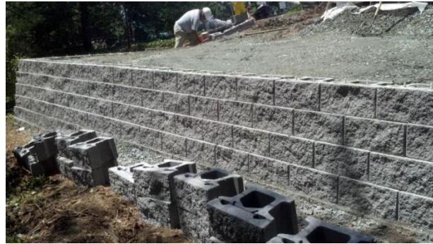
Figure 7: POB Parking Construction, Photo Taken By: Brandon Tezak
