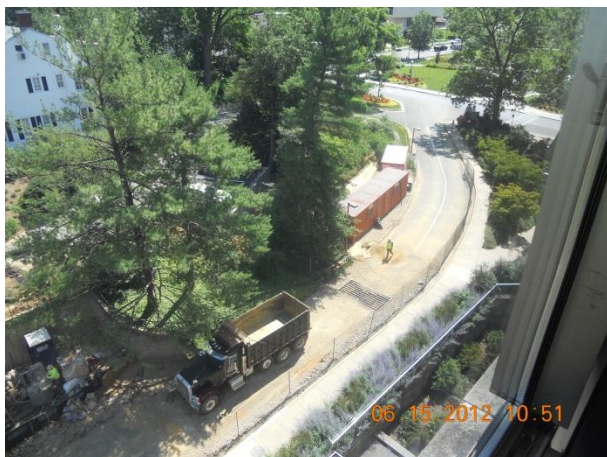
Figure 10: North Hall Site Entrance, Photo Taken By Brandon Tezak
