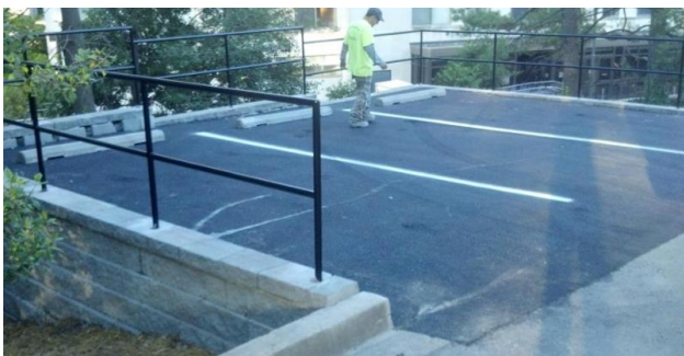
Figure 8: POB Parking Complete, Photo Taken By Brandon Tezak
